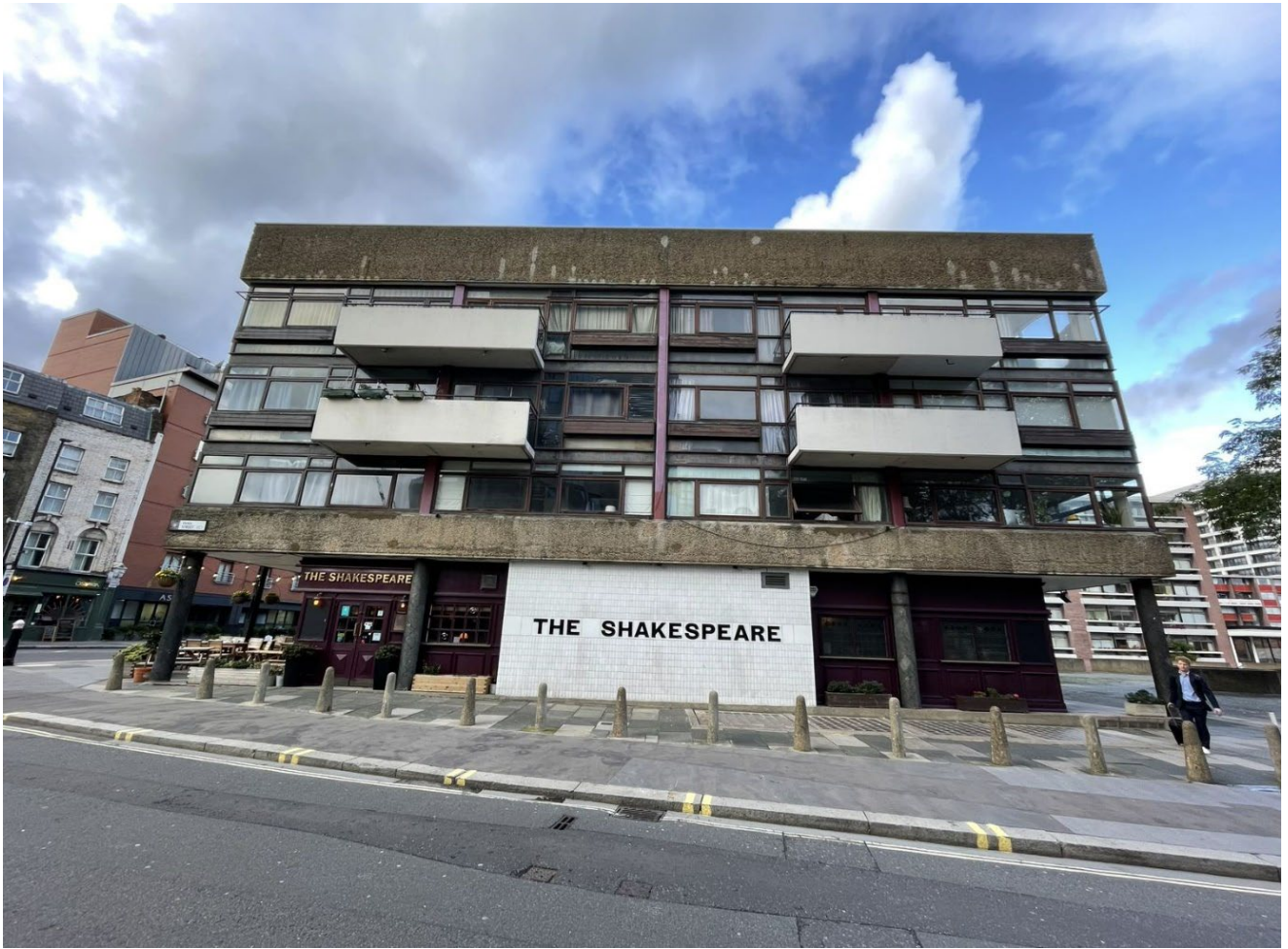
Image 3 – Crescent House, Southern Elevation (facing Fann Street)
