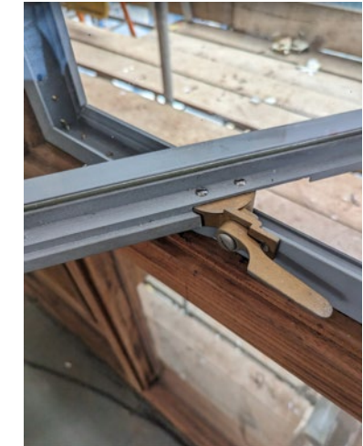
Existing window with VIG installed
