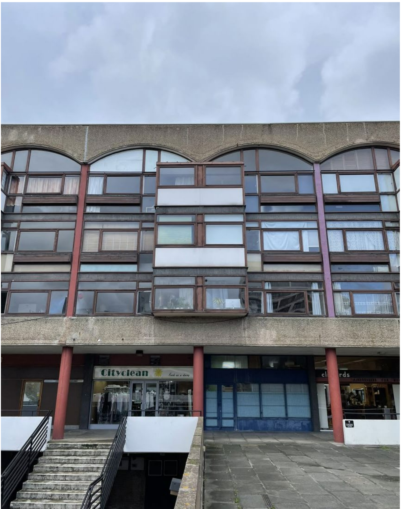
Image 2 – Crescent House, Eastern Elevation
