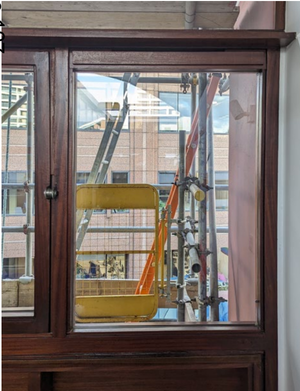
Internal view of trickle vent
