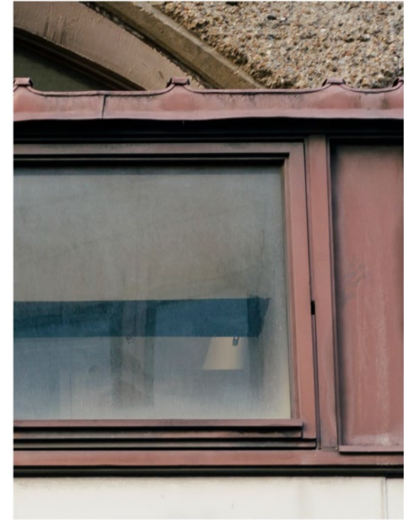
Original Window – no obvious rot
