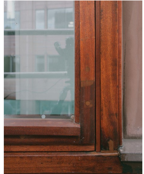
Completed repair, window reinstalled and oil finish applied
