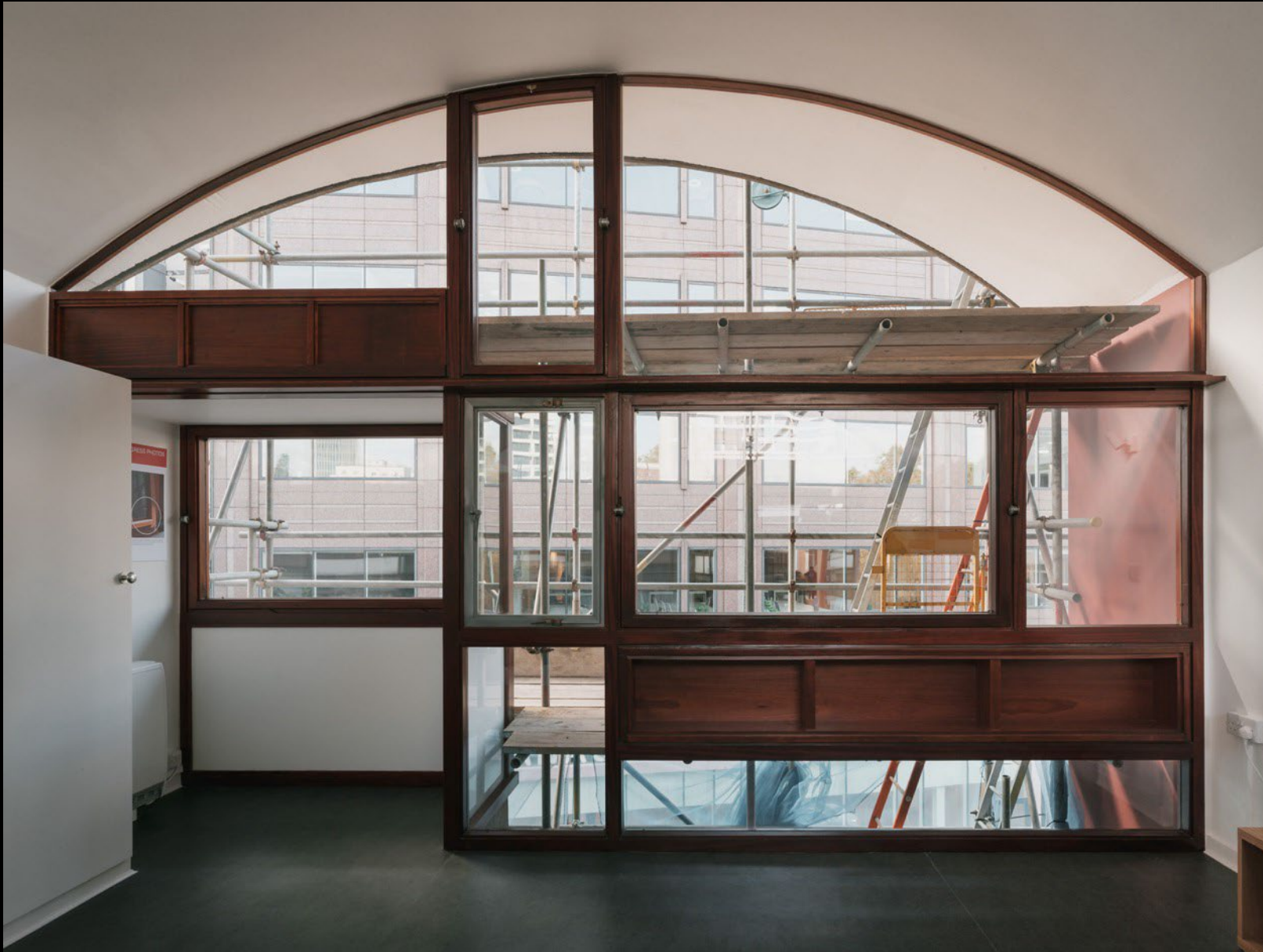
Interior of 347 Crescent House after completion of Pilot Project
